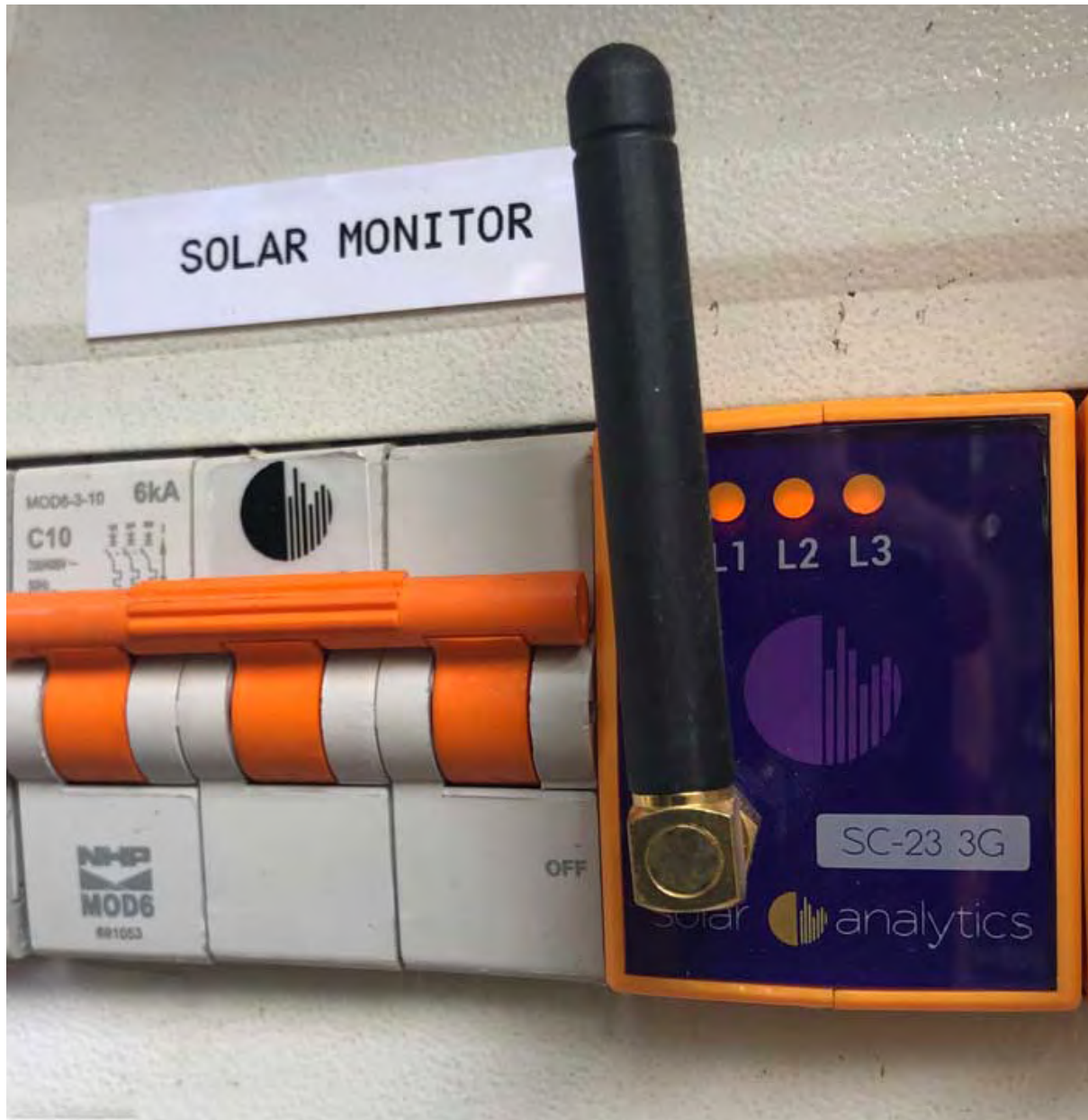
A consumption monitor in my switchboard.
