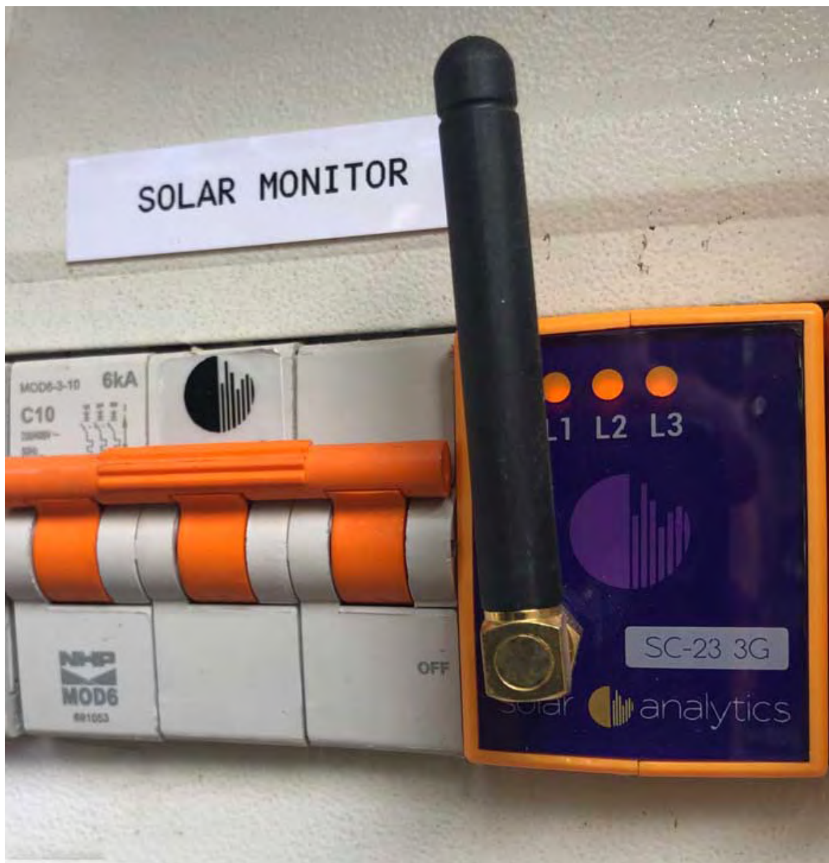
A consumption monitor in my switchboard.
