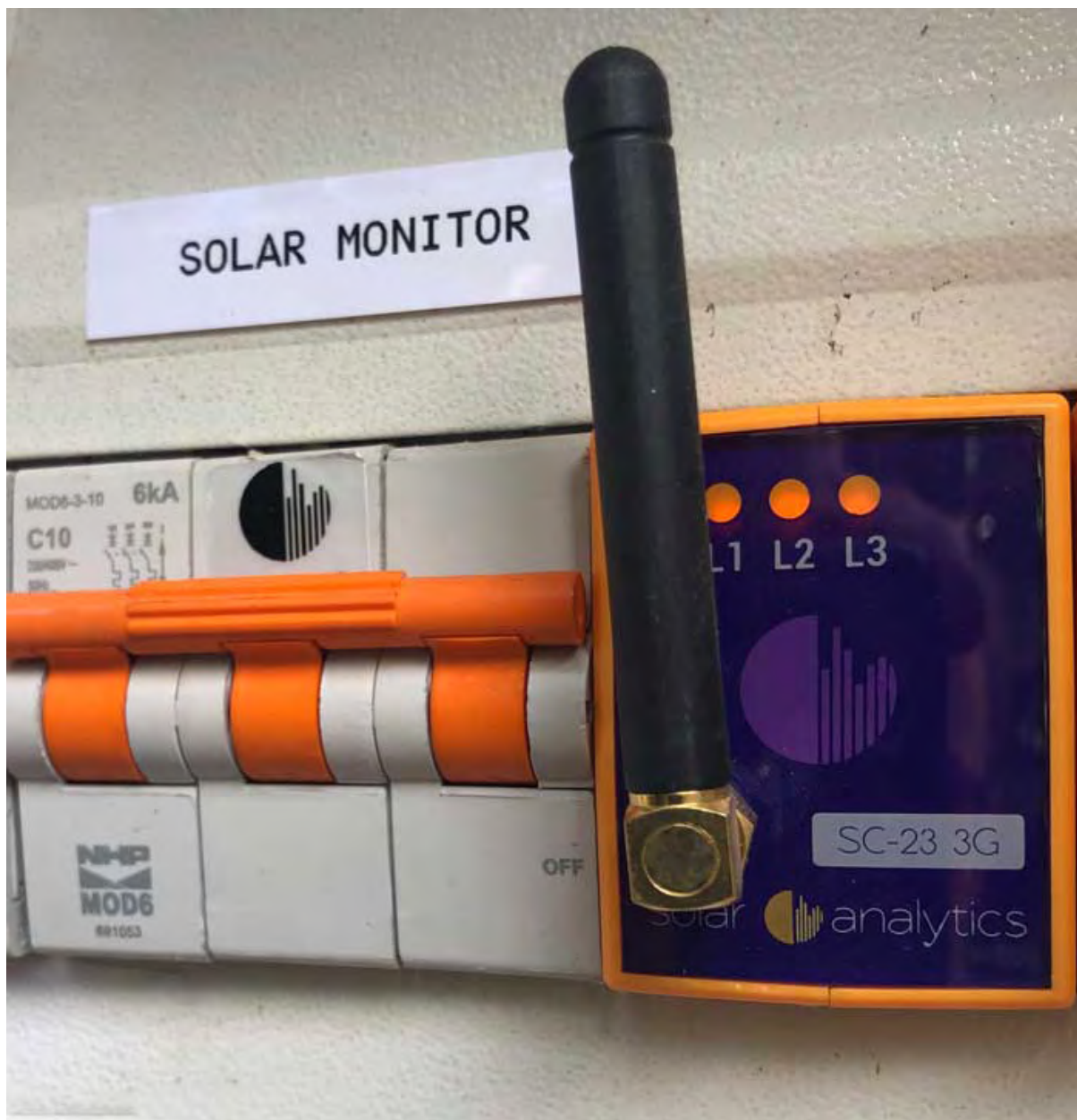
A consumption monitor in my switchboard.
