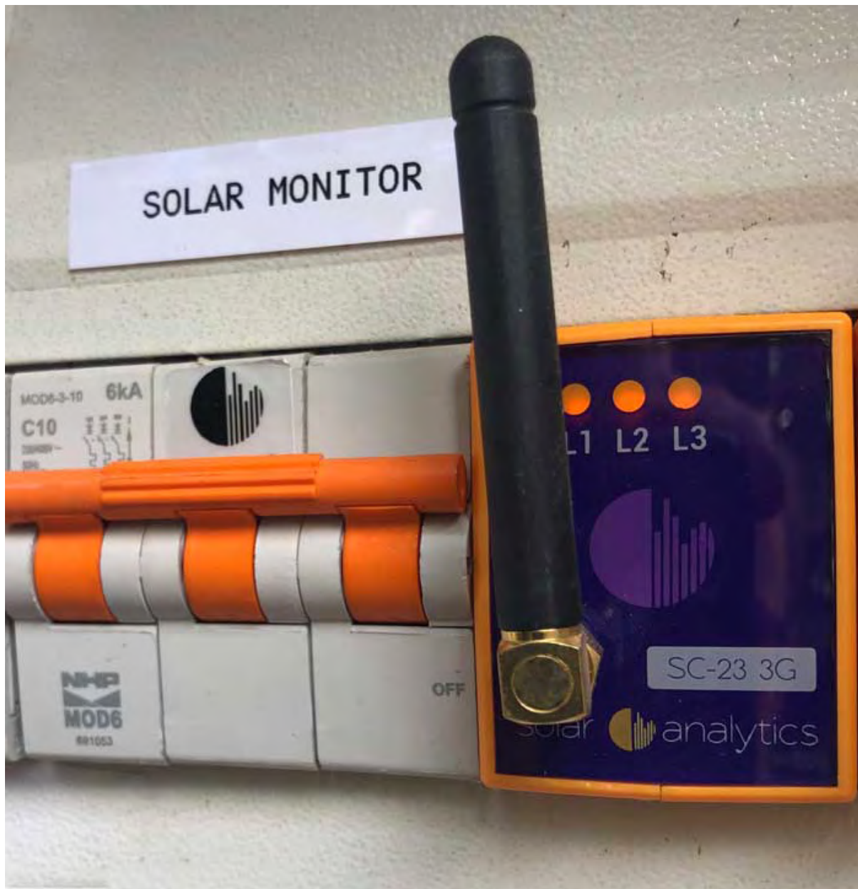
A consumption monitor in my switchboard.
